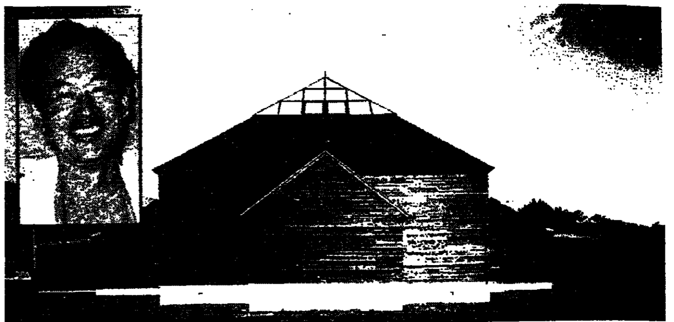
Architect Arata Isozaki's barnlike building outside Tokyo, the latest museum of contemporary art founded by Toshio Hara, inset.
